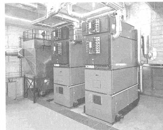
Figure 5.8: Two 3,2 MWth inclined moving grate furnaces for wood chips, used for district heating in Interlaken (Courtesy of Schmid AG, Switzerland).
