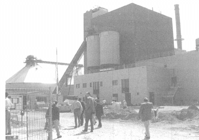
Figure 5.17: A 25 MW e woodchip-fired power plant in Cuijk, The Netherlands, with a BFB boiler.
