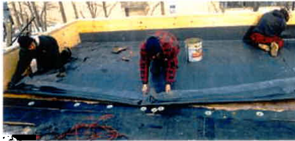
Figure 2. After the adhesive has tacked up, workers roll the EPDM into place (top). Wrinkles are smoothed out with a stiff bristle broom (bottom).
