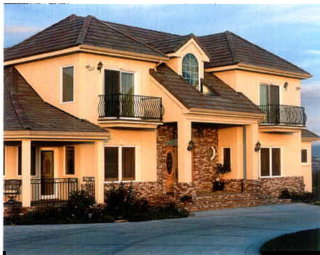
You can't tell from the street. Vinyl windows have moved into the upper end of the residential market. In this new Los Angeles home, only the door is wood.
