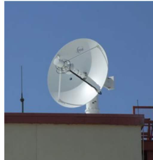
A newly installed antenna sits atop the U.S. Air Force Test Pilot School. The antenna is part of a new aeronautical telemetry ground system that will allow airborne data to be transferred to the ground in the C-band frequency range – an addition to the L- and S-band frequency ranges currently used. The new tri-band system will increase bandwidth and allow more frequencies to be used by both the civilian community and Edwards Air Force Base. (Courtesy photo)
