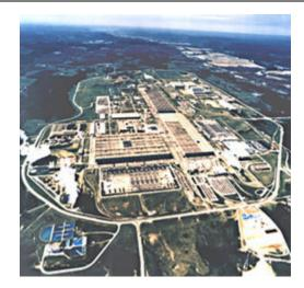
Relies on molecular effusion (the flow of gas through small holes) to separate U-235 from U-238. The lighter gas travels faster than the heavier gas. The difference in velocity is small (about 0.4%). So, it takes many cascade stages to achieve  $e^{235}UF_{6}$  even LEU.
