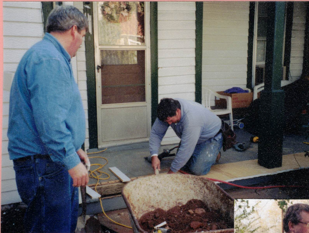
mike, Enos + marty do an amazing repair job on the front porch!
