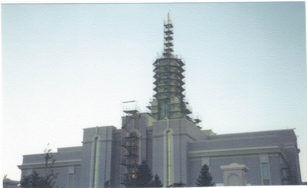
Mt. Timpanogas Temple being repaired.
